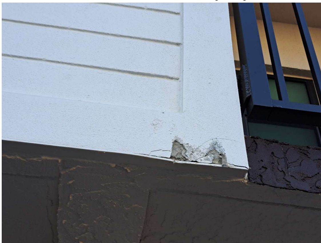
Photo 04 Ref: 2.1.1.1 – Stucco & Siding Damage
