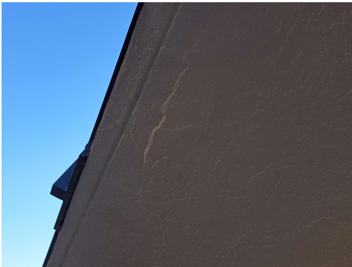
Photo 09 Ref: 2.1.1.1 – Stucco & Siding Damage
