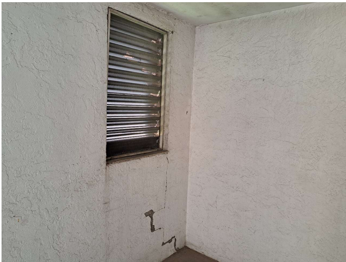
Photo 14 Ref: 2.1.3.1 – Debonded Stucco and Cracks in Louvered Corner Rooms
