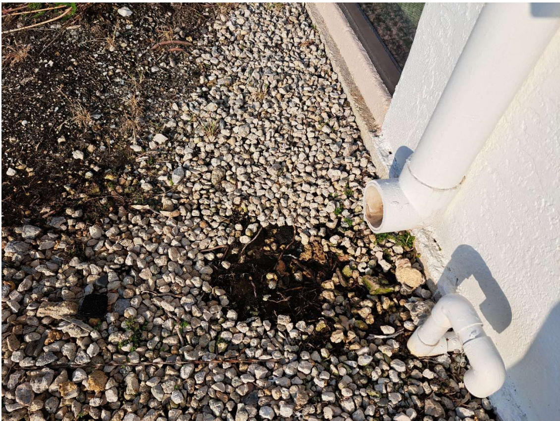
Photo 11 Ref: 2.1.2.1 – Downspouts Emptying Next to Foundations
