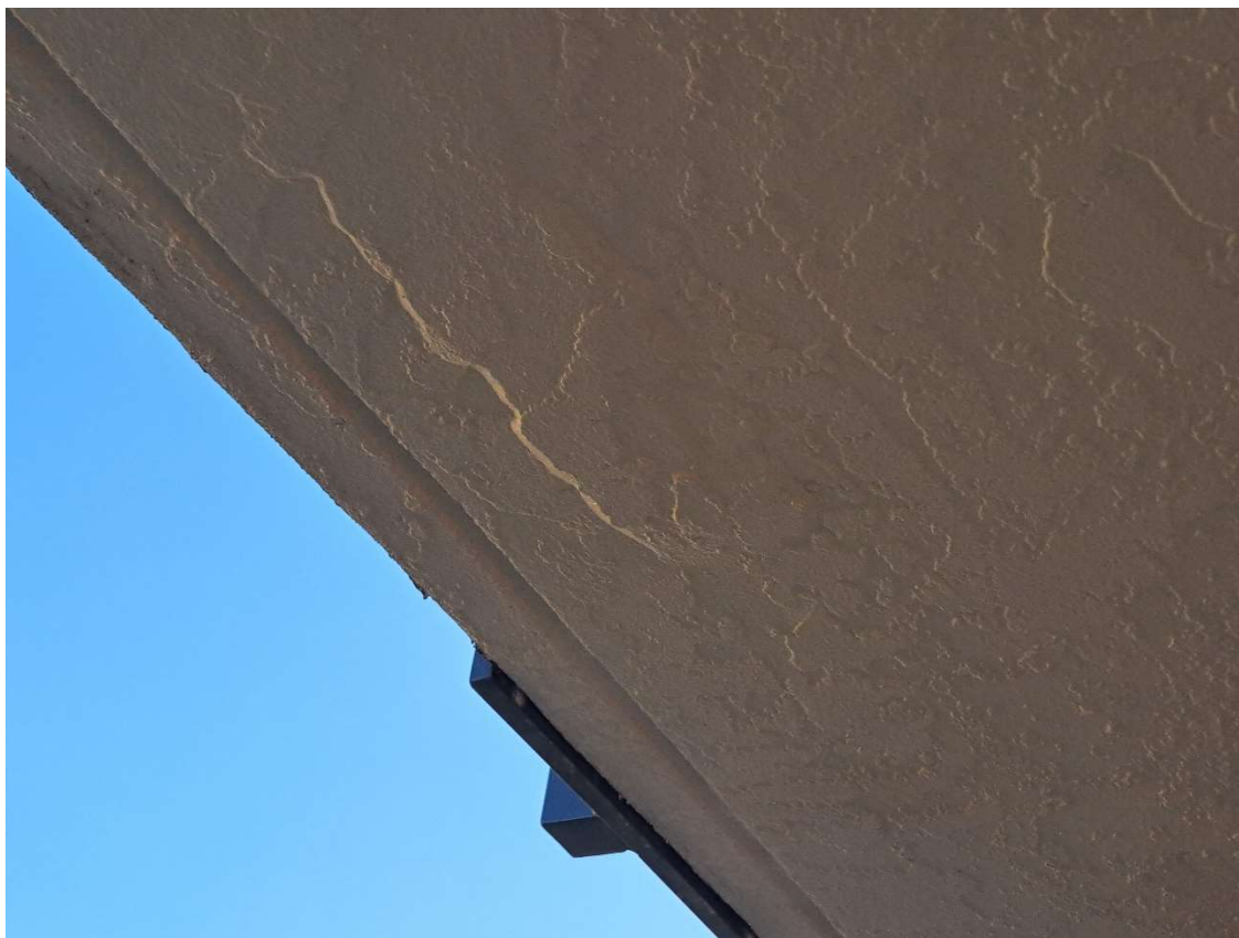
Photo 10 Ref: 2.1.1.1 – Stucco & Siding Damage
